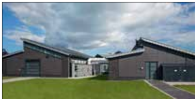
Laboratory and technical centre facilities of ISF SCHAUMANN RESEARCH
